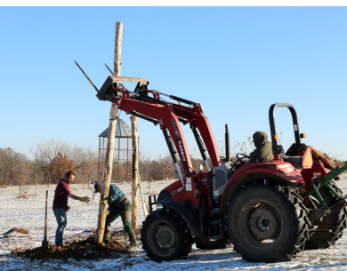
Installing black locust poles.
